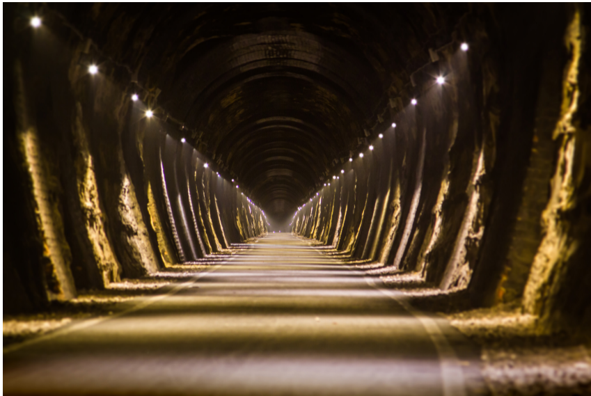
Combe Down Tunnel (length 1.6 kilometres )
